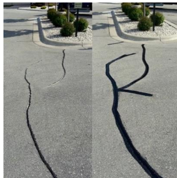
Fig 17- Crack repairing using Self-Healing material
