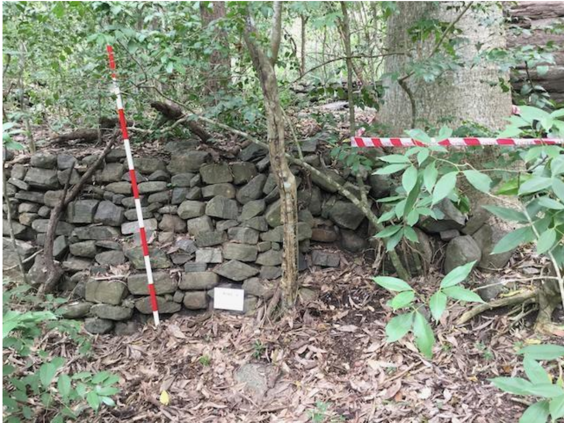
Figure 25: this image is showing a very big tree (Ebony ( diospyros sp) ) and smaller ones growing around. This particular dry-stone terrace wall cannot be saved but be left to its fate since the big tree cannot be fell.
