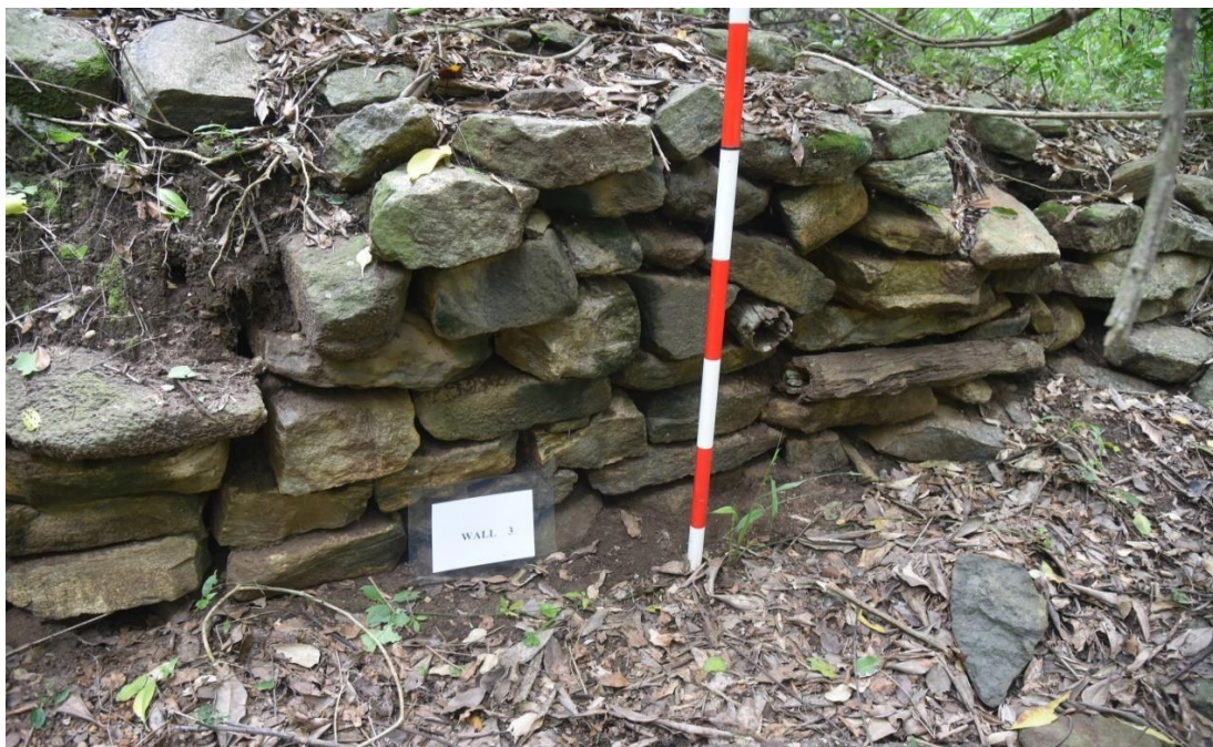
Figure 4: A picture of a terrace wall in the shape of a rectangle with height of 0.9 metres. (Photograph by Miss Odarkor Ankrah-Addison, July, 2020).
