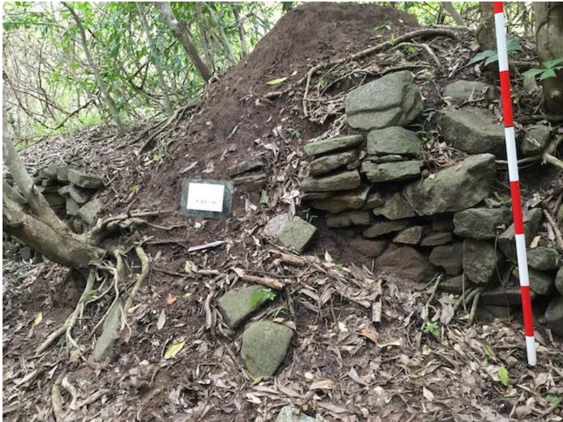
Figure 26: even though in this picture there is a presence of a tree, the ant hill built on top of the terrace wall is also adding up to the destruction of the wall.
