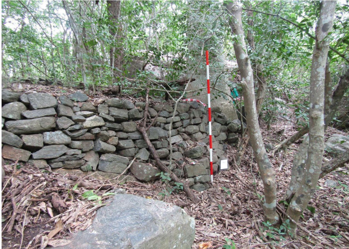
Figure 15: This picture shows the wearing out of the dry-stone terrace walls due to a big tree growing by its side causing the roots to penetrate through the wall (Photograph by Miss Odarkor Ankrh-Addison, July, 2020).
