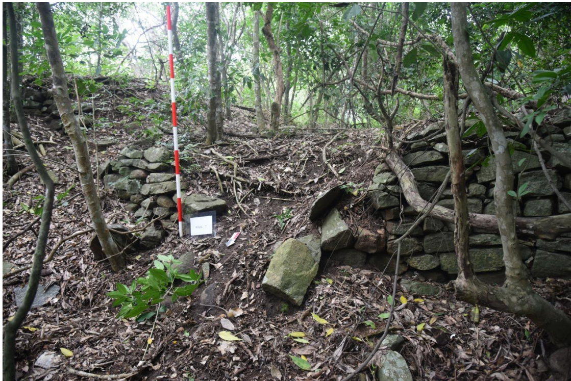
Figure 11: A picture showing how roots and branches of trees pulling and falling stones from their original position to the ground (Photograph by Miss Odarkor Ankrah-Addison, July, 2020).
