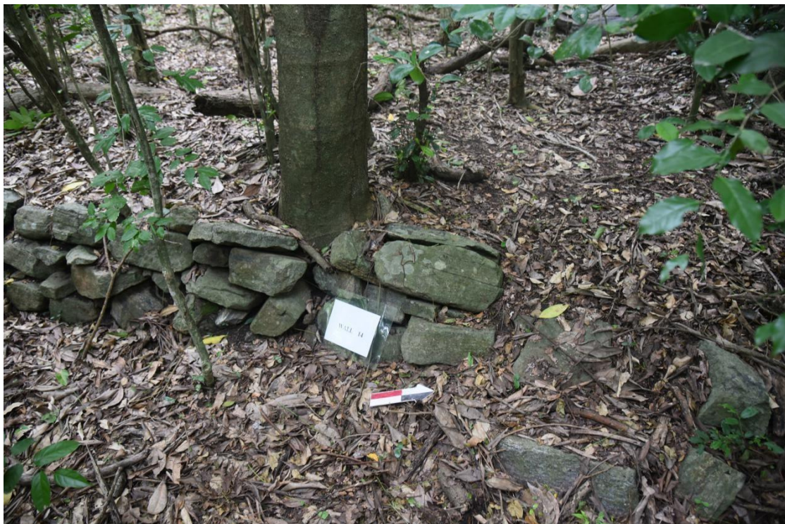
Figure 13: Another picture showing how the roots of trees outside of the terrace pulling down the stones of the terraces (Photograph by Miss Odarkor Ankrah-Addison, July, 2020).
