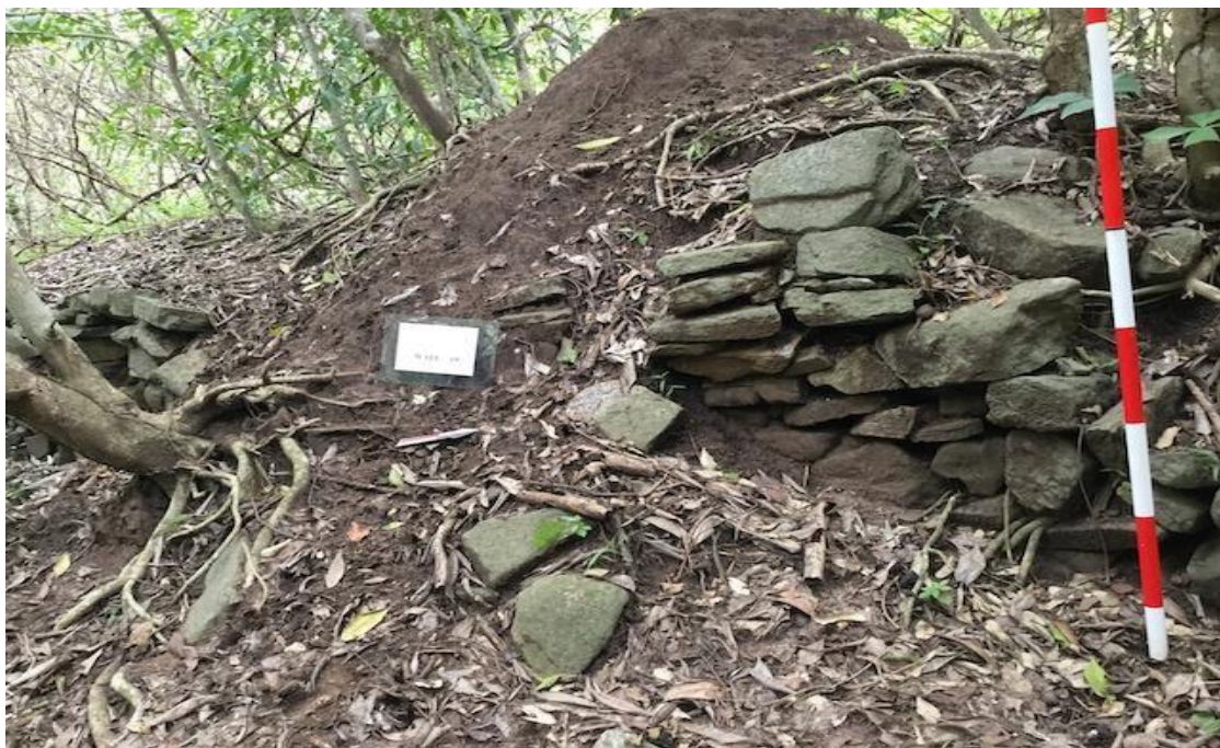
Figure 23: this picture is showing a tree growing in front of a terrace wall and its root causing havoc to the wall. This wall can be saved by felling this tree and removing all of its roots that are penetrating though the walls (Photograph by Miss Odarkor Ankrah-Addison, July, 2020).
