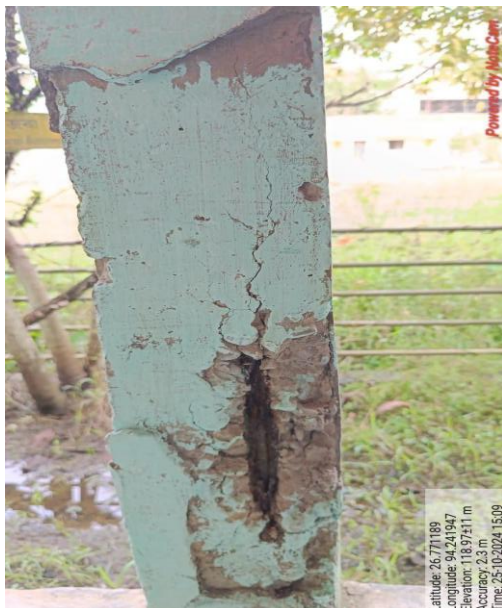
Fig 18.3 : Crack on post
