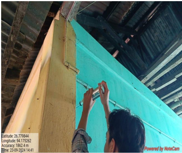
Fig 6.3: Performing Rebound Hammer Test
