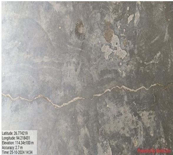
Fig.17.3: Crack on floor
