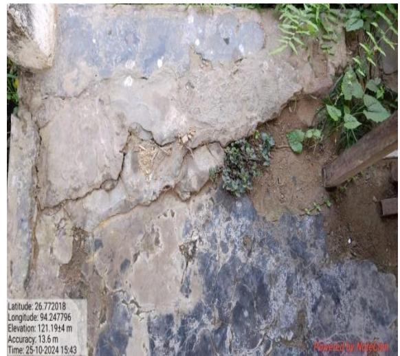
Fig 20.2: Crack on wall
