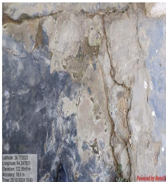
Fig 20.3: Crack on floor
