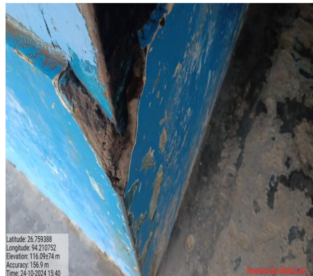
Fig 14.2: Crack on wall
