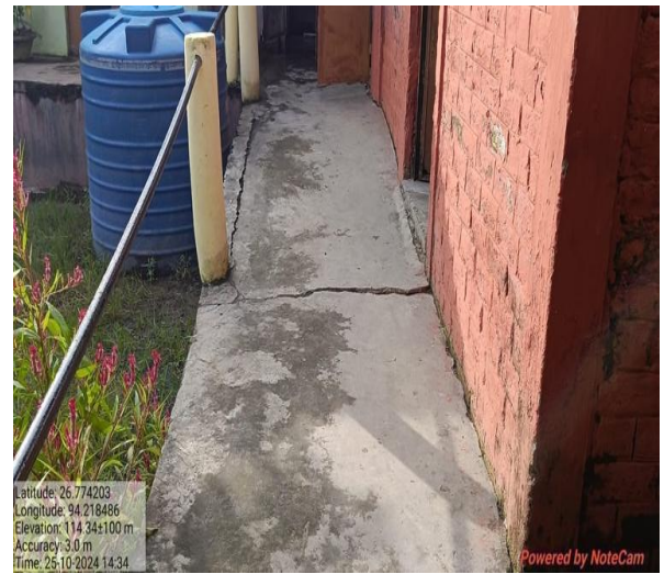
Fig.17.4: Crack on ramp
