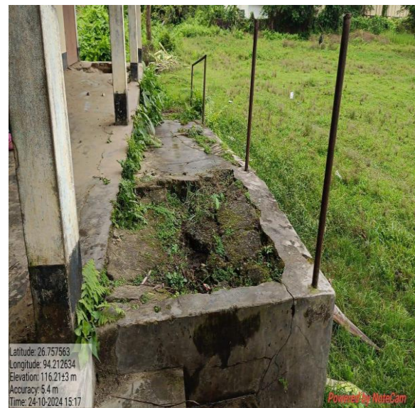
Fig 12.4 : Crack on ramp
