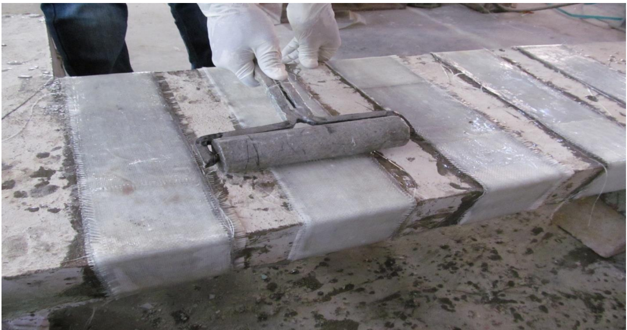
Fig 3.6 Roller used for the removal of air bubble
