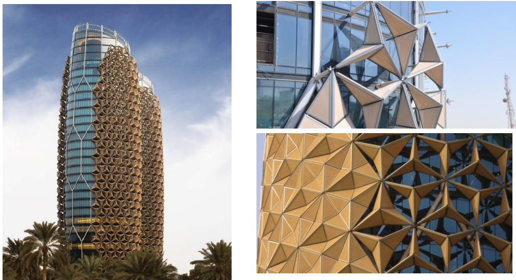
Figure 7. Al Bahr Towers And Dynamic Facade
