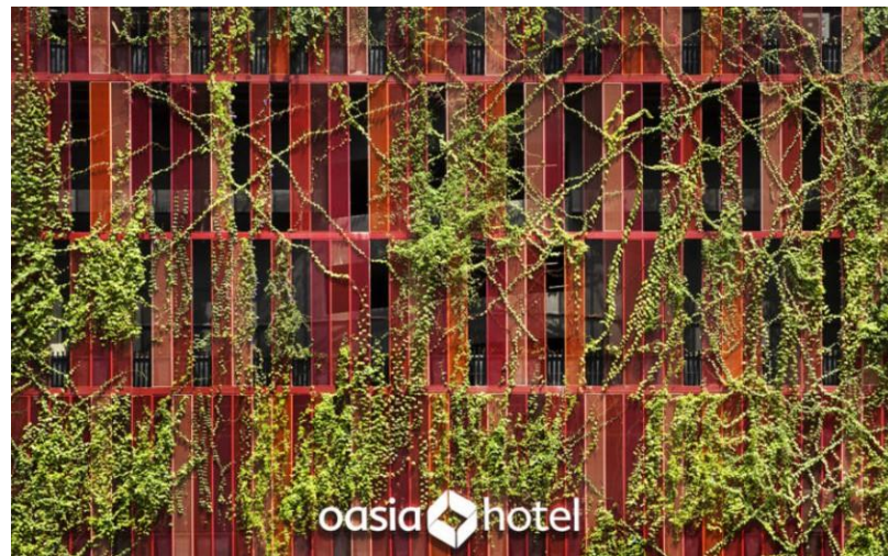
Figure 12. Green Facade With Mesh And Plants
