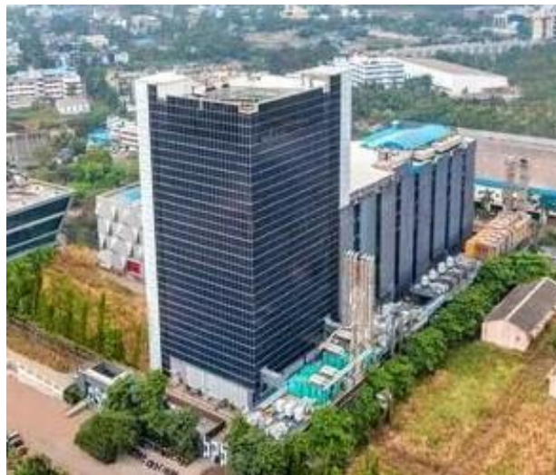
Figure 10. Ctrl's Dc2 Data Centre
