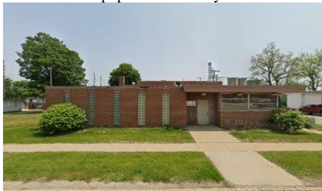
Fig. 1. The Central Office for CenturyLink in LaGrange, Indiana
