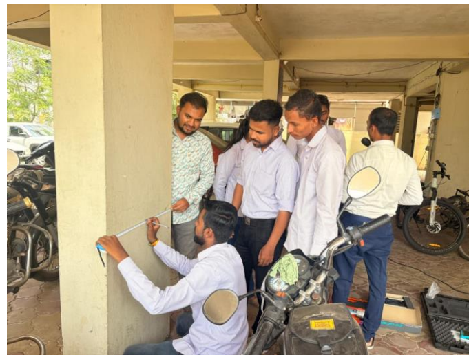
Fig. 4. Field investigation in progress — Rebound Hammer and Rebar Locator testing on a column
